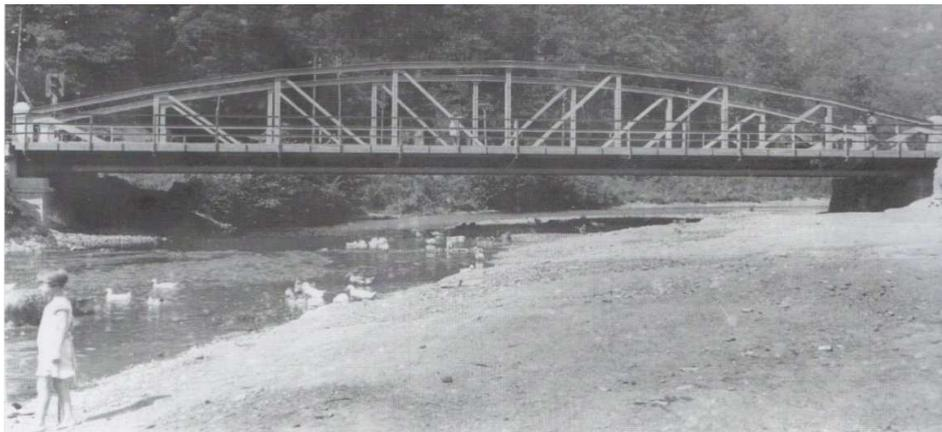
**Figure 6** The first welded bridge mounted across the Bârzava River at Stavila
