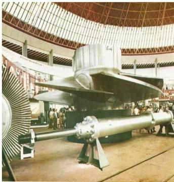
**Figure 16** The Kaplan rotor
