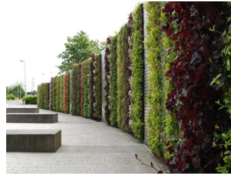
Figure 3. Indirect green facade
