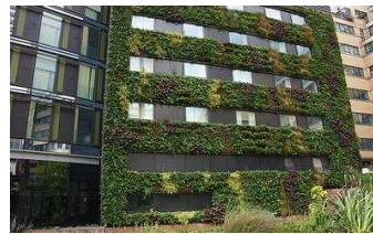
Figure 5. Modular living wall system
