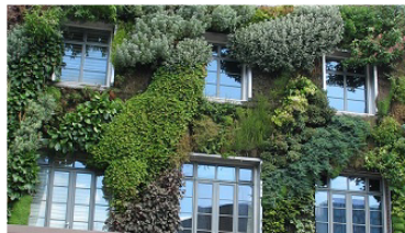
Figure 4. Continuous living wall system
