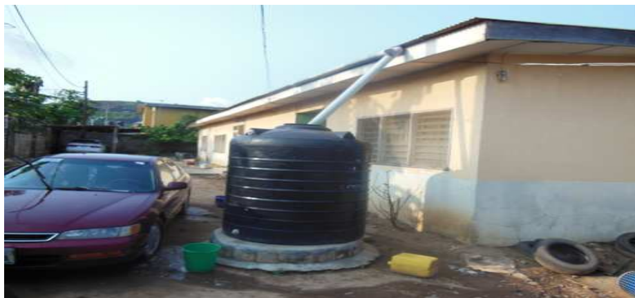
Plate 1. Rainwater harvest from surface roof plan
