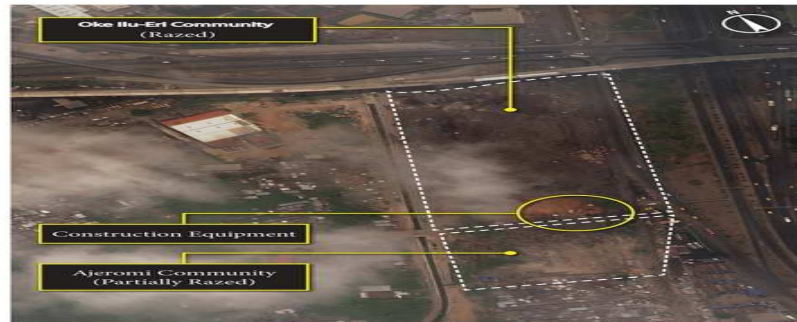
Figure 5. A satellite image of Badia East after demolition Source: bigstory.ao.org
