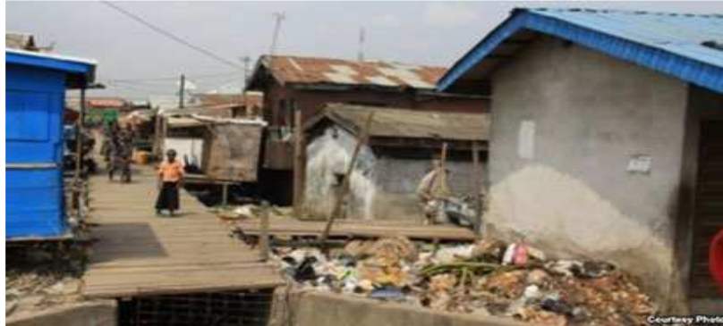
Figure 2. Building condition of Badia East before demolition Source: bigstory.ao.org
