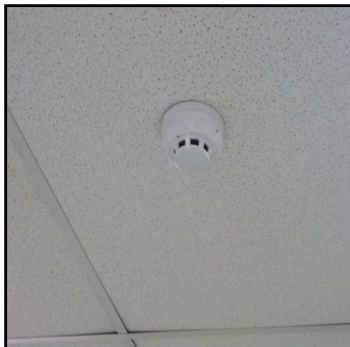
Figure 1. Common type of smoke detector found in the market.
