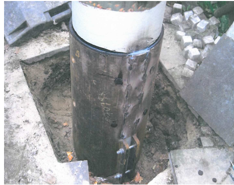
Figure 5. Pipe with sleeve, assembled /3/
