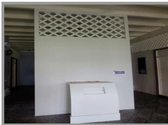
Figure 6. Timber structure covered with "Papan Lapis Cantik" material
