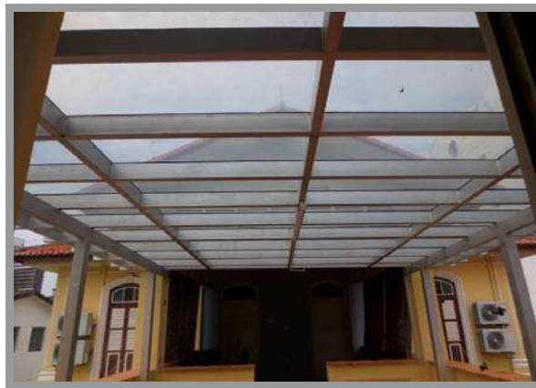
Figure 8. Sun shelters at the first floor area
