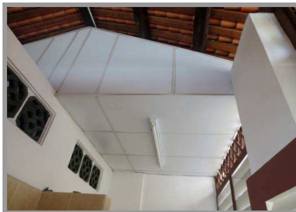
Figure 9. Suspended ceiling in the toilet
