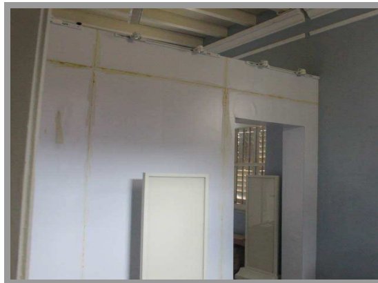
Figure 5. Addition of partition wall at the ground floor
