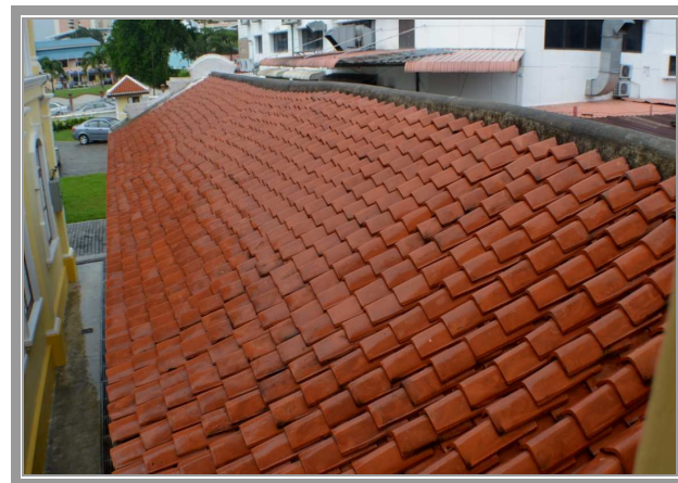
Figure 18. Replaced V tiles for roof covering
