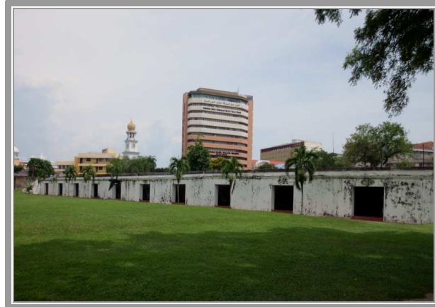
Figure 23. The cell rooms
