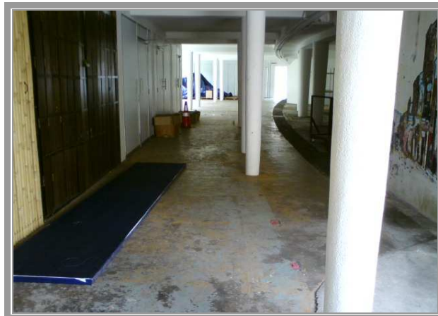
Figure 21. The columns that react as support structure
