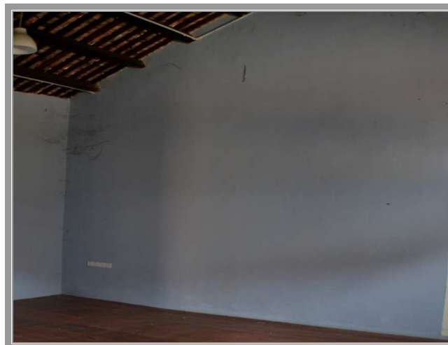
Figure 15. The interior wall paint for Rumah Teh Bunga
