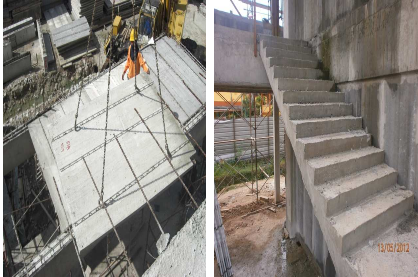
Figure 7. Examples of half slab and stair installed on site
