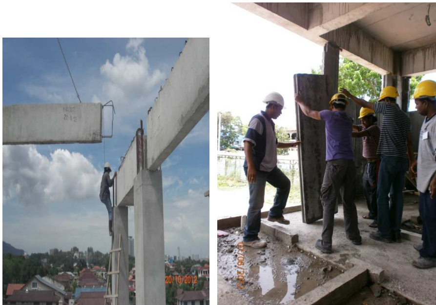
Figure 8. Examples of wall panel and beams installed on site
