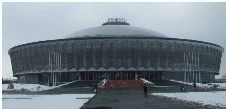
Figure 2. General view of the building
