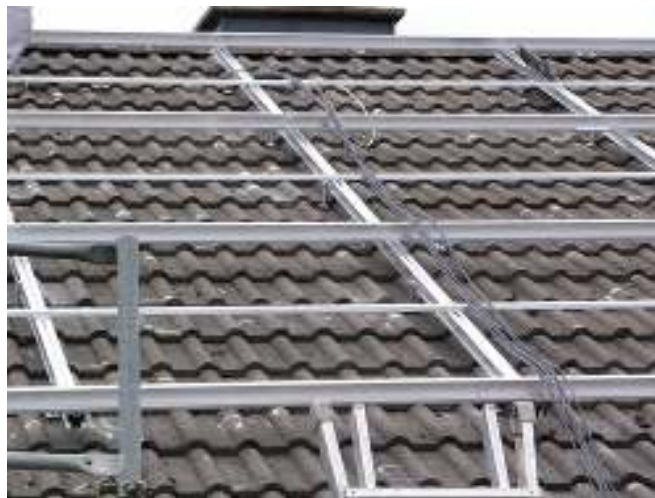
Figure 2. Settlement schemes of solar modules on the roof of the building
